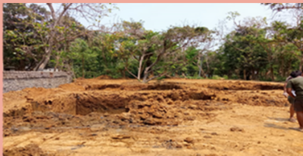
Excavation of land for AS
