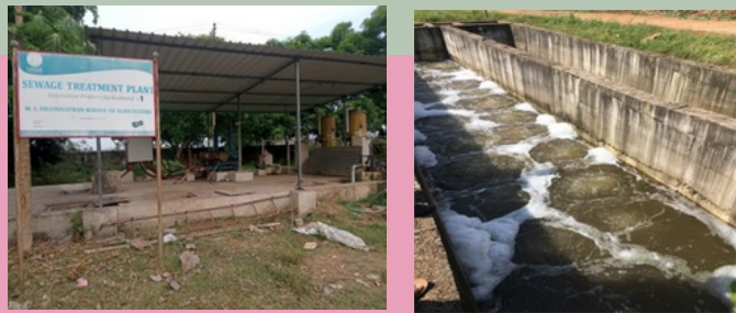
Sewage Treatment Plant (STP)
