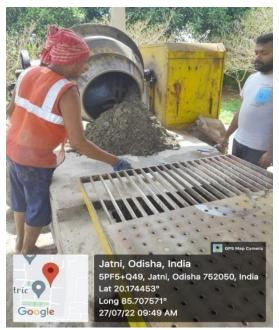
Figure 5 Removing of wet mix for pouring to block mould
