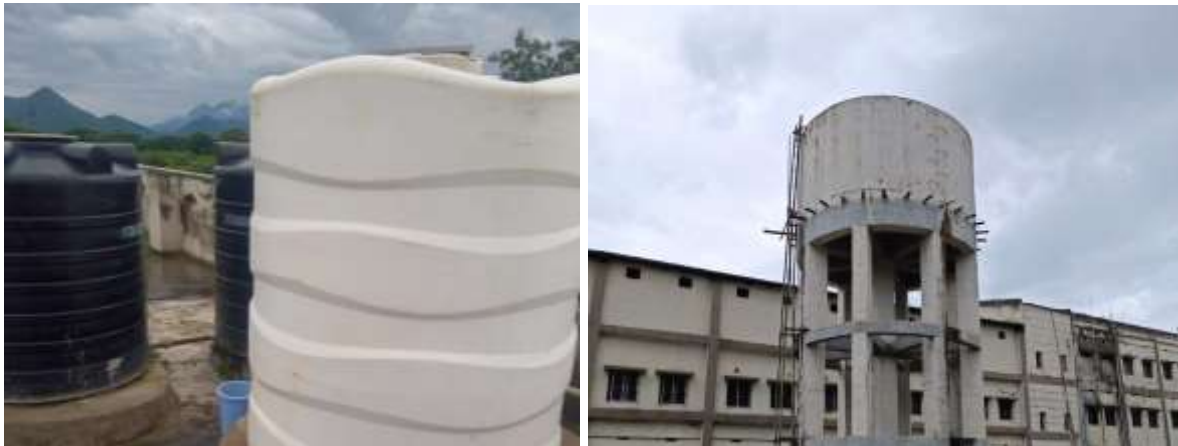
Figure: 1.4- Image of Overhead Tank
