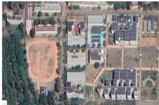
Satellite view of Grid Connected Roof Top Solar System
