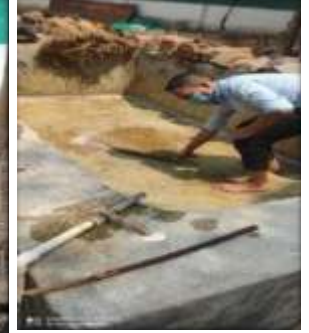
Clearing of tank for soaking
