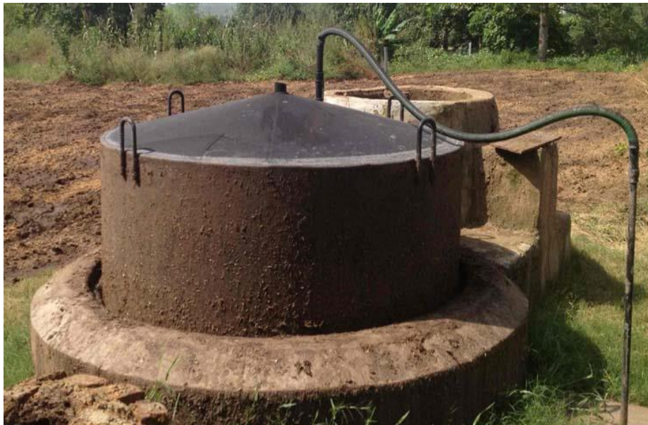
Fig: Food waste and cow dung digester (Biogas plant) for generation Biogas in tribal village,
