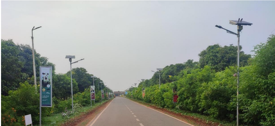
Fig. 3 shows the solar power street lights in Centurion University campus.
