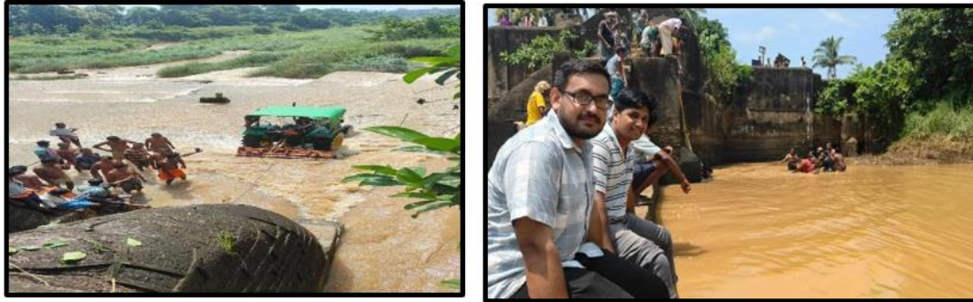
Figure 7: Cleaning of canal for irrigation
