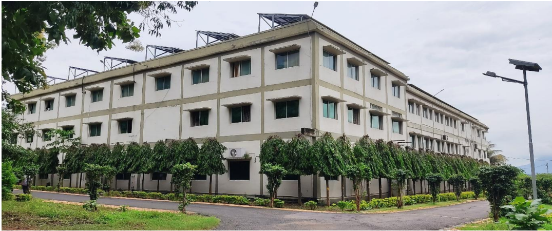
Solar Panels Fixed in the top of the Main Building at Centurion University
