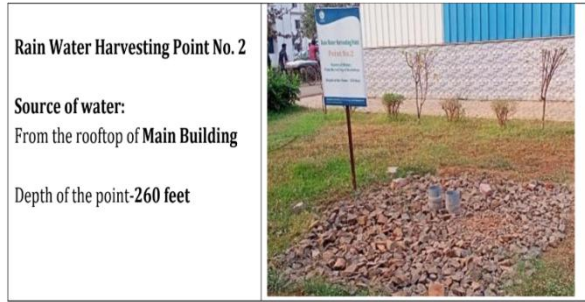
Rain Water Harvesting Point-02
