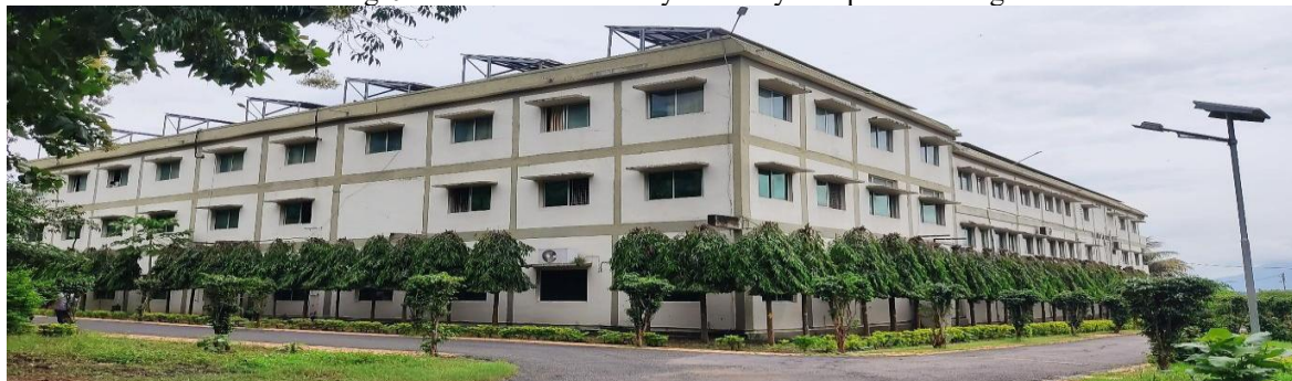
Fig-02: Solar Panels Fixed in the top of the Main Building at Centurion University
