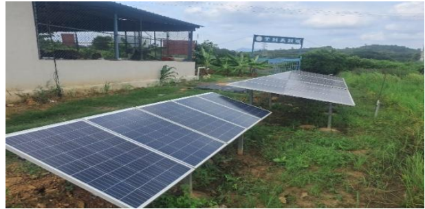
Fig:-08 Micro-Grid at Centurion University
