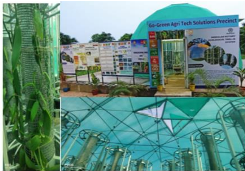
Fig.99 Automated Polycarbonate-based Polyhouse & Polyhouse at PKD Campus
