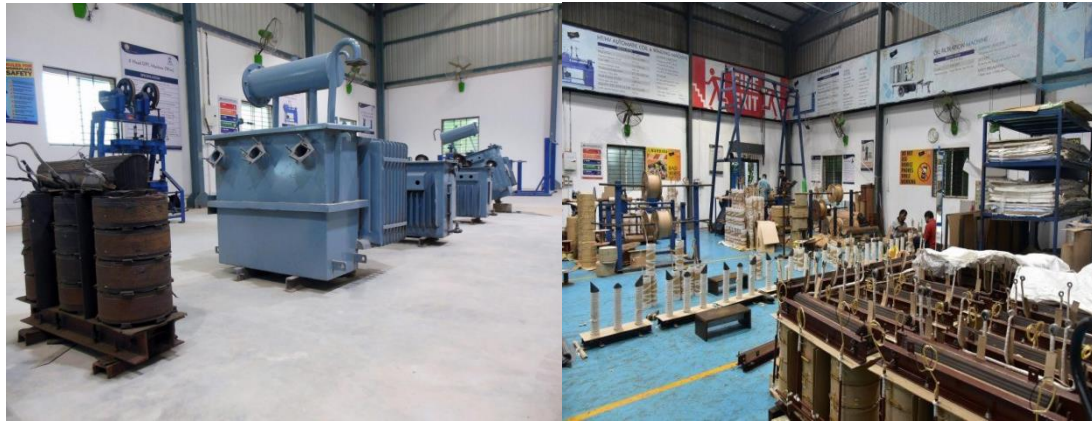
Fig.33 Different Types of Machine in Tranformer Unit
