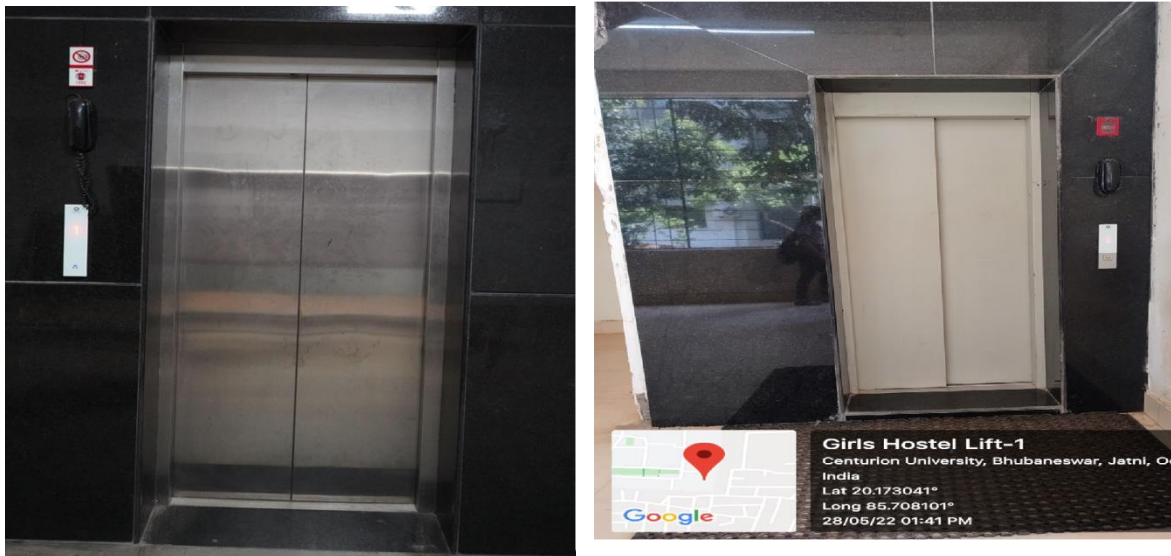
Image 7.4: Elevator in the Hostel building and Management Building
