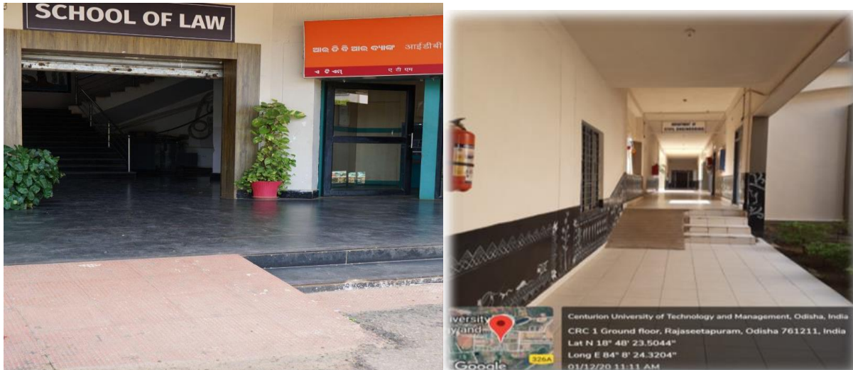
Image 7.2: Ramps in the Management building
