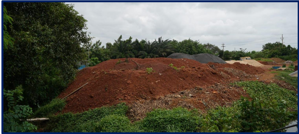
Fig. 27 Construction and demolition wastes utilized for in-campus land filling
