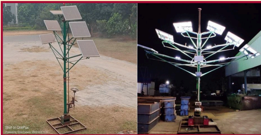
Solar Power Plant
